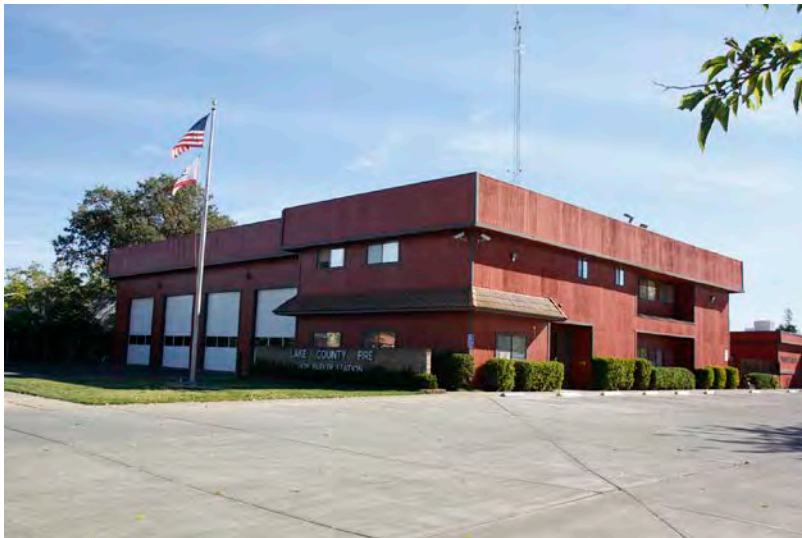
Cal Poly Land Use Inventory, 2012. Clearlake Fire Station
