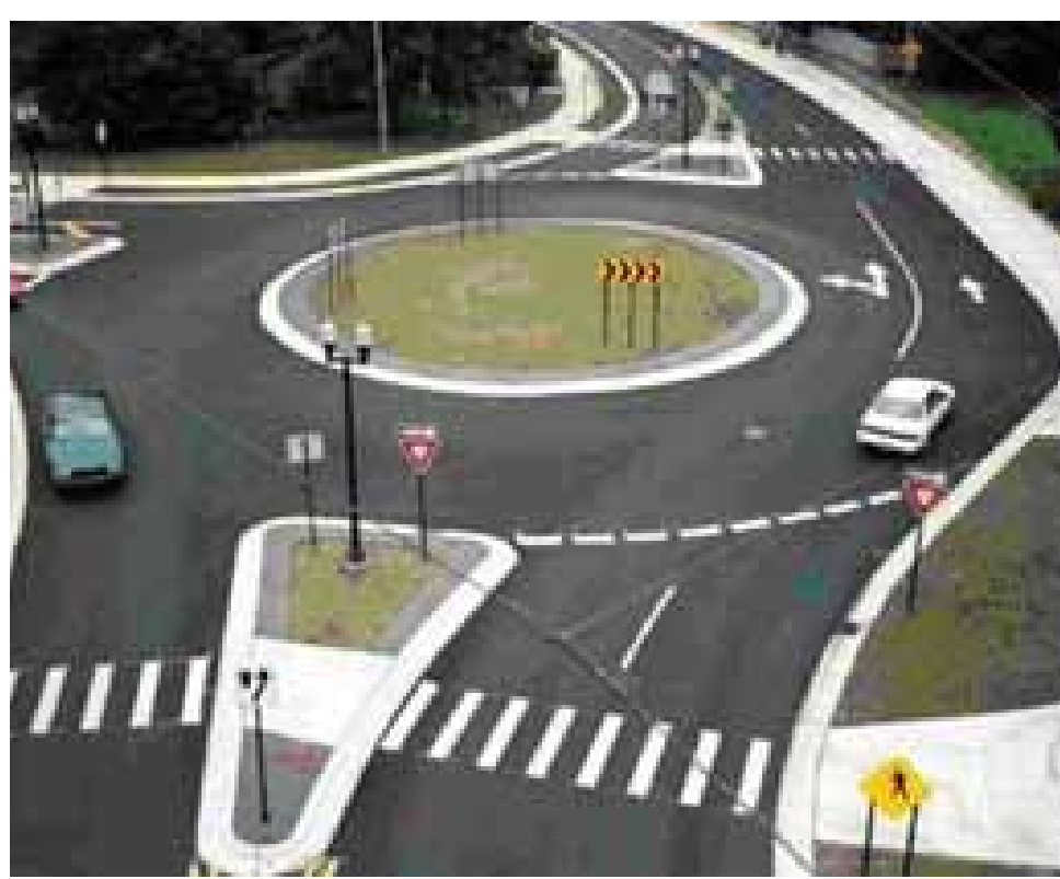
Traffic calming to restrict vehicular speed
